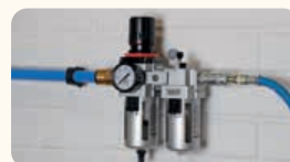
FILTER/REGULATOR/LUBRICATOR
